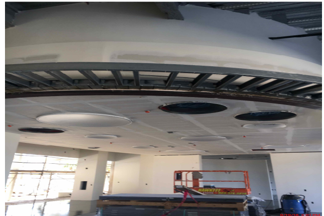
Building T1 Interior
