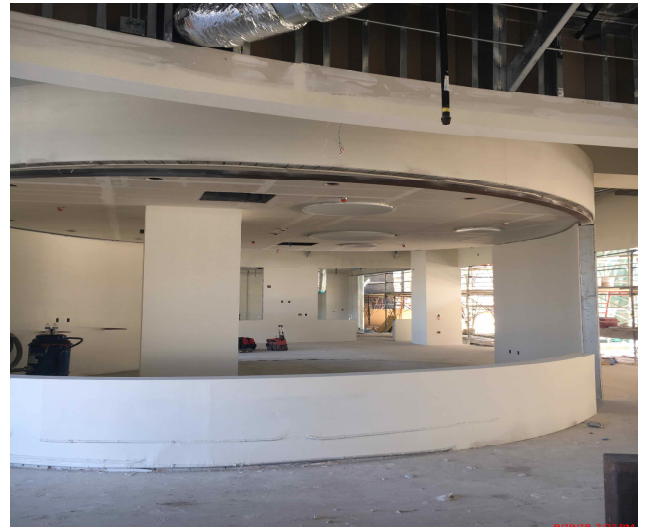
Building T1 Interior
