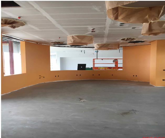
Building T1 Interior
