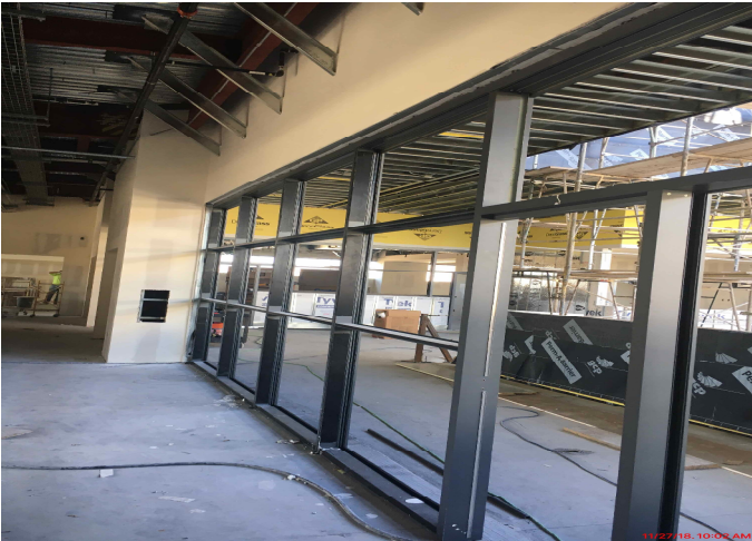
Building T2 Interior
