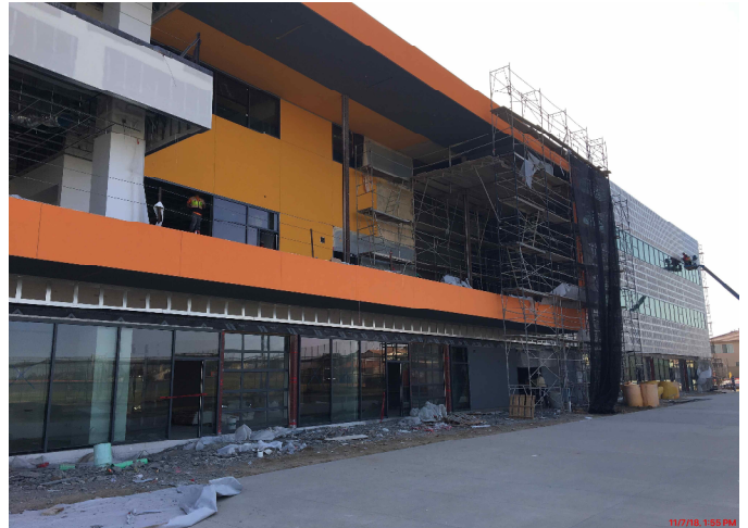
Buildings T1 Exterior
