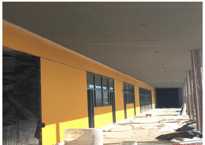
Building T1 Exterior
