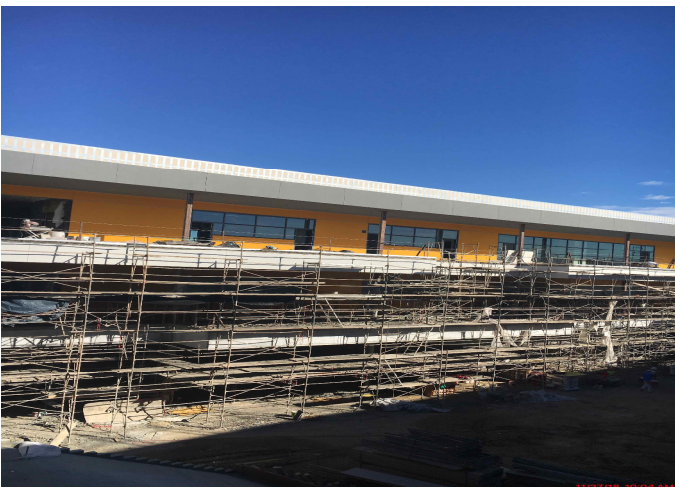
Building T1 Exterior
