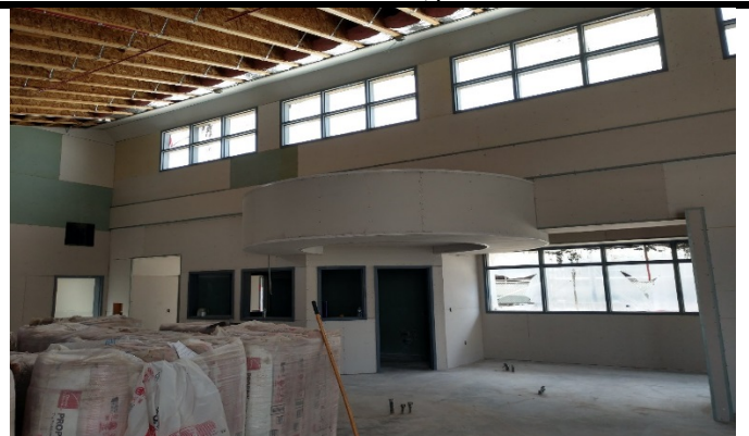
Building C drywall
