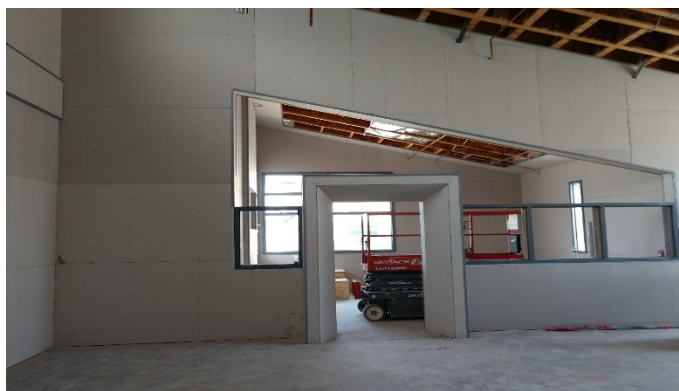
Building C drywall at Story Room
