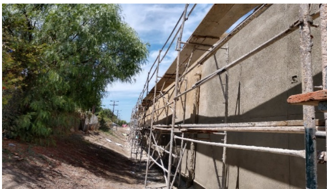
Building D Stucco color coat at rear of building
