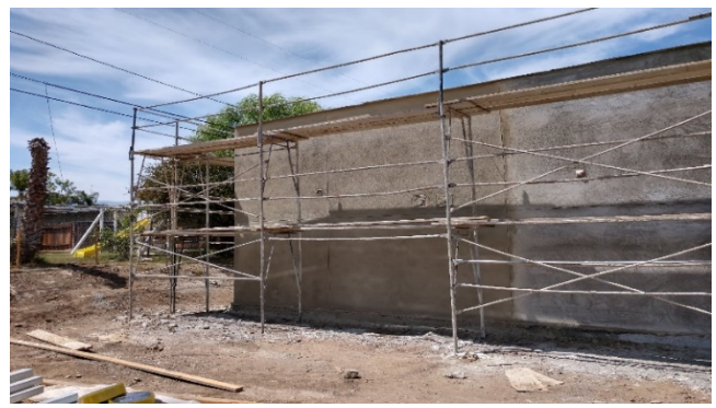
Building D stucco color coat at front of building
