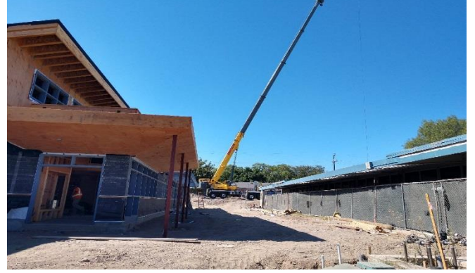
Setting HVAC Equipment Both Buildings
