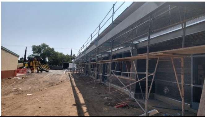
Finish scaffolding and lathing Building D
