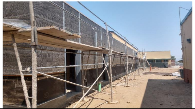
Finishing Scaffolding @ Building C
