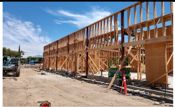
Wall Framing @ Building D
