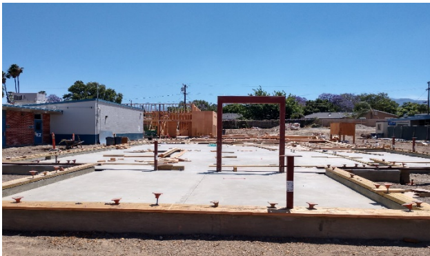
Plate walls Building C
