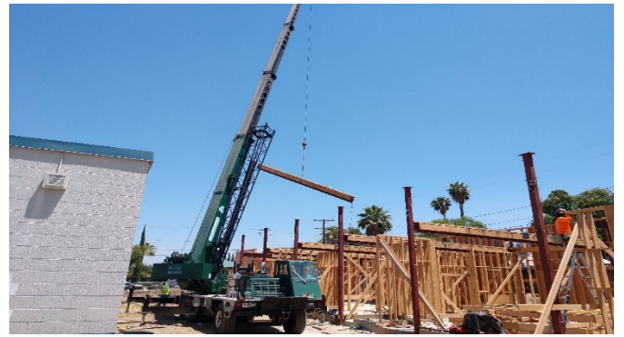
Setting steel @ Building D
