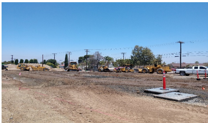
Site work , Parking lot Grading
