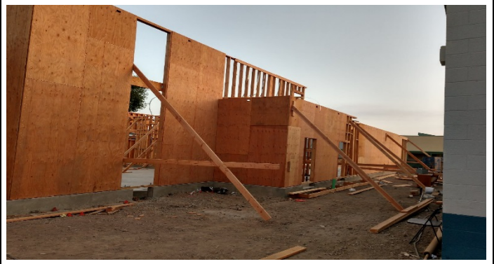
Framing Walls Building C
