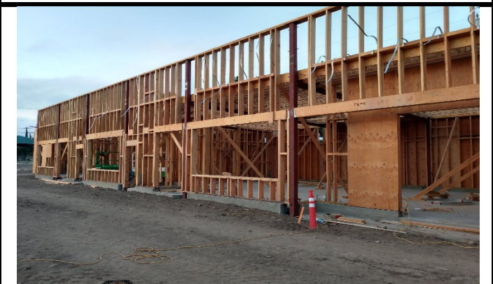
Building D , Wall Framing
