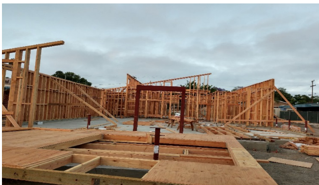
Framing Walls Building C
