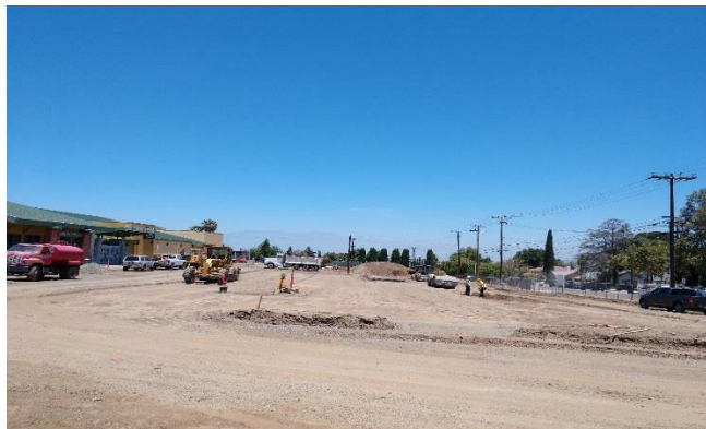
Site work, Parking lot Grading
