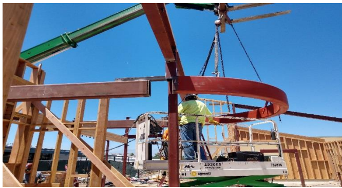
Setting Steel Building C
