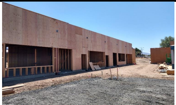
Building D, Sheeting complete
