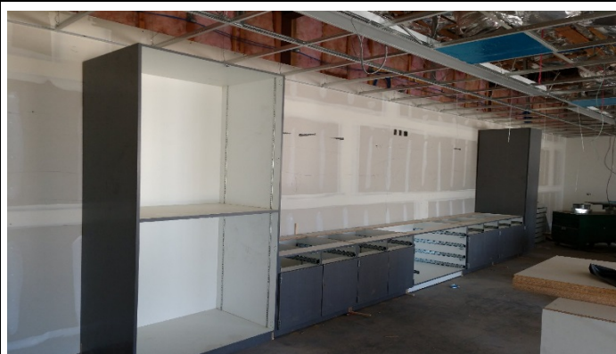
Casework in progress at building D
