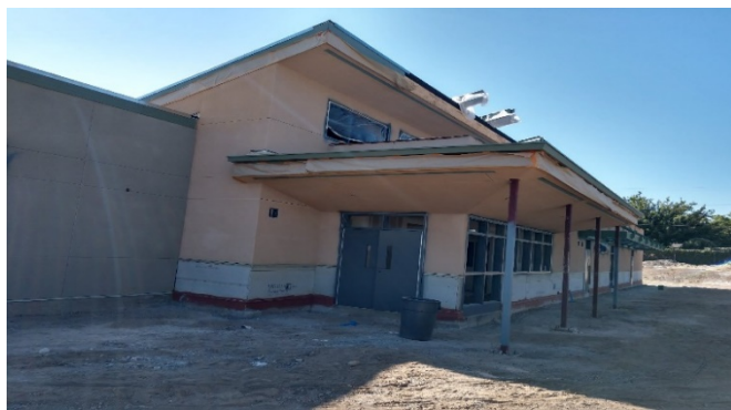
Building C exterior painting
