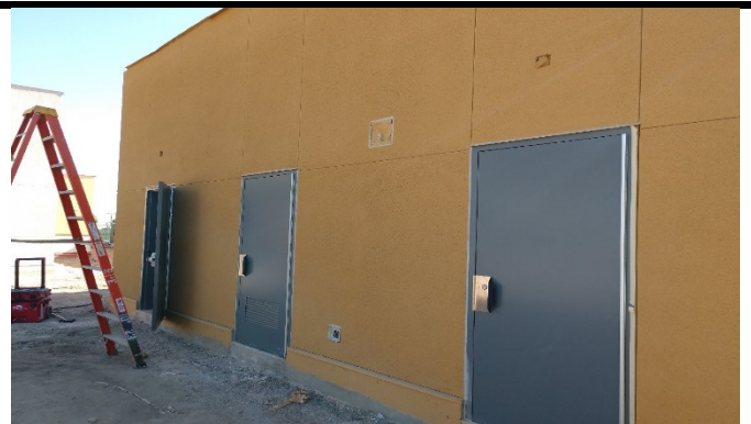
Building D Door Installation
