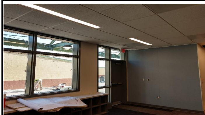
Building D, Casework in Progress
