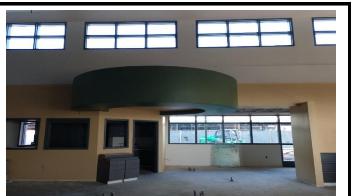
Building C, Paint complete
