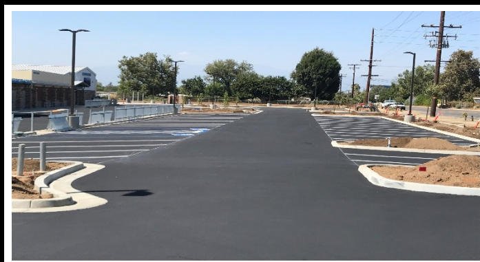
Parking seal coat & striping
