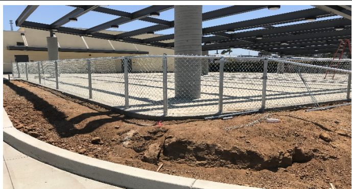
Chain link fence
