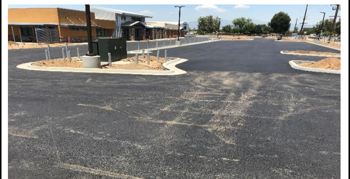
Parking lot asphalt
