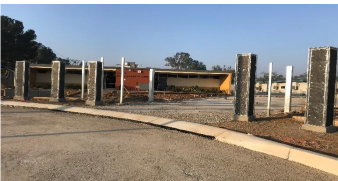
Lath on block columns
