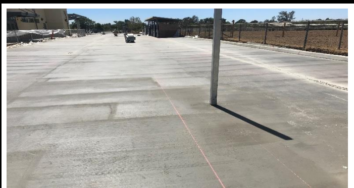
Fire lane concrete
