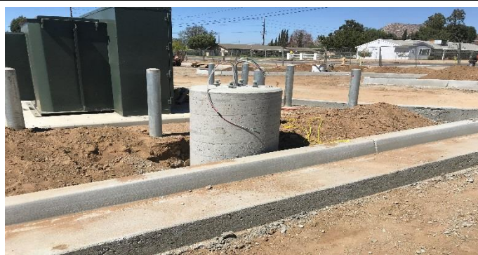
Light pole base
