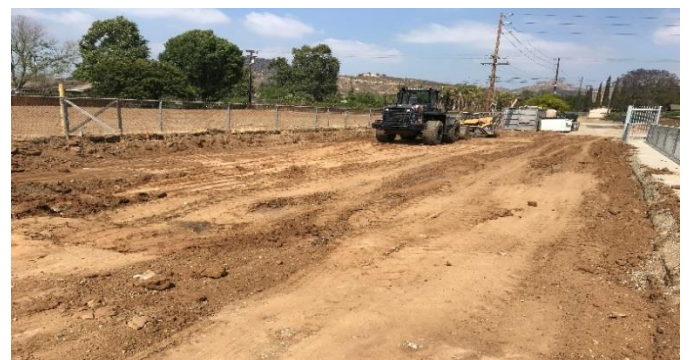
Fire lane grading
