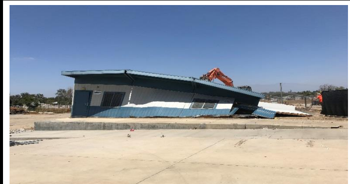
Old Library demolition
