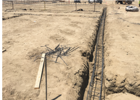
Area's A-D Rebar Installation
