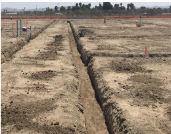
Area's F&G Footing Excavation
