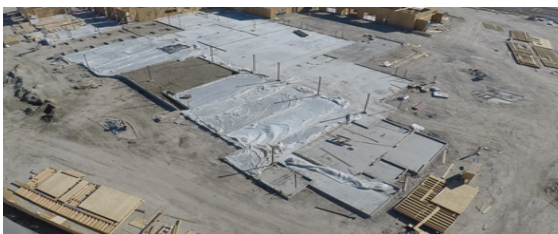
Area F-G Slab
