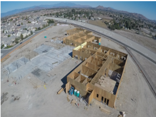
Area E Framing
